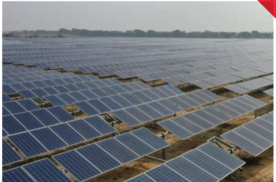
Groundmounted Solar System - Merino Rohad (H.R.)
