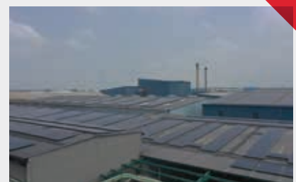
Rooftop Solar, MIL Rohad
