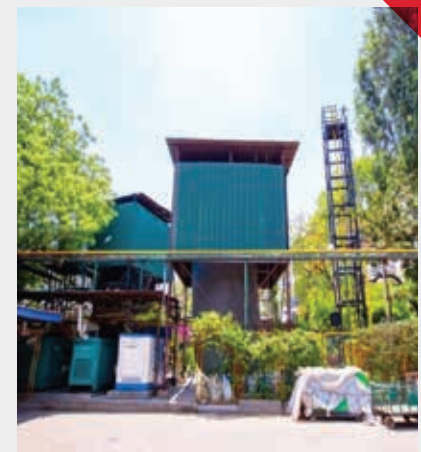
Biogas system, MIL Hapur
